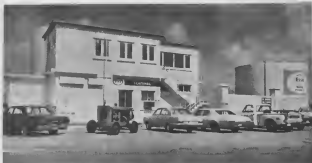
The second floor has been added to the Oranjestad Terminal building to provide space for the new Esso Marketing Office.
